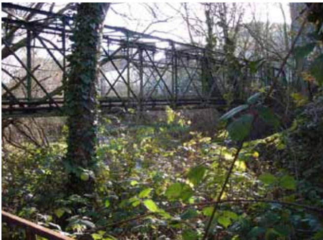
The Bishops Mill pond and the cable bridge before works were carried out
