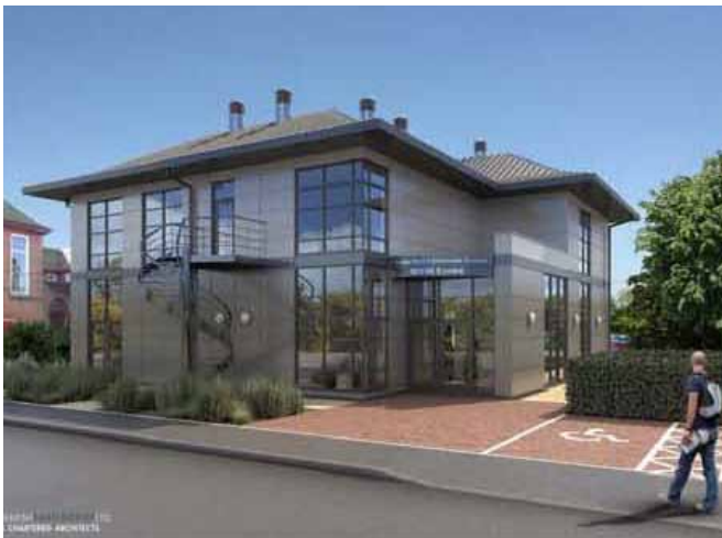
Main Entrance - Rear Elevation
